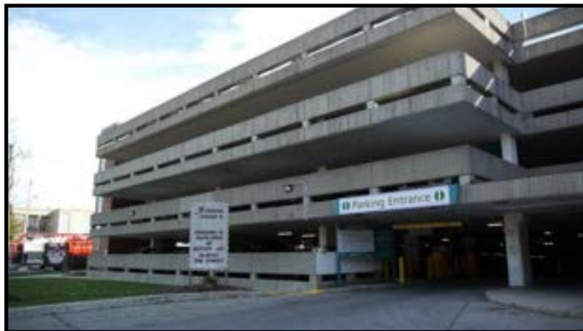
Main Parking Garage on 835 King St. West.
